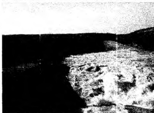
15.2 - rasm. Qiyshiq gidravlik sakrash oqibatida inshoot pastki befini yuvilishi.
