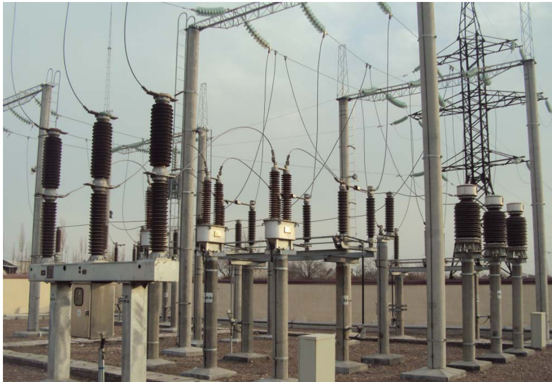
70-rasm. 110 kV tashqi o'chirgichlar.
