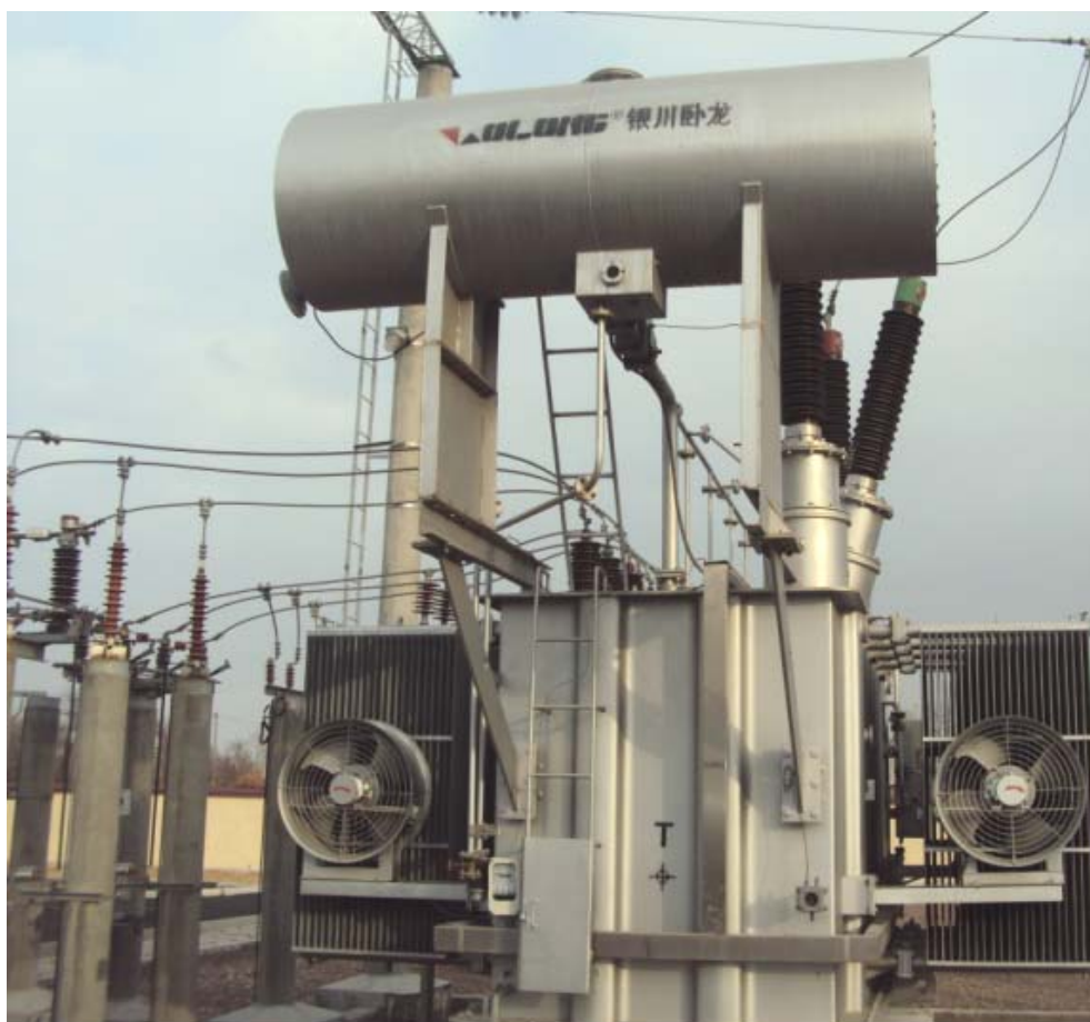
66-rasm. Kuch transformatorining sovitish tizimi.
